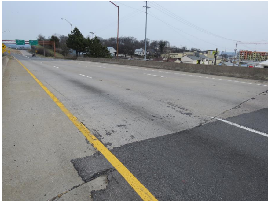
VIEW ACROSS TOP OF WEARING SURFACE
