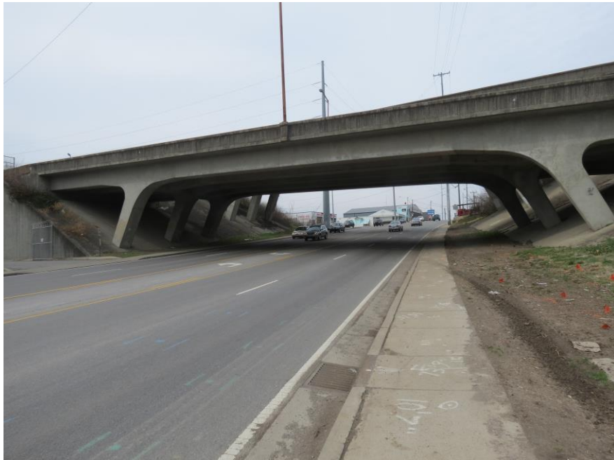
CLEARANCE VIEW LT. SIDE
