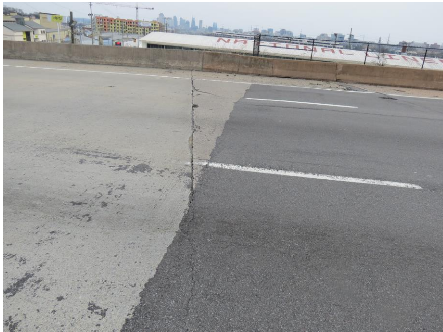
APPR. "B" END JOINT PAVED OVER
